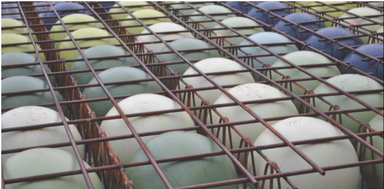
Figure 27: Voided concrete slab configuration before concrete placement
